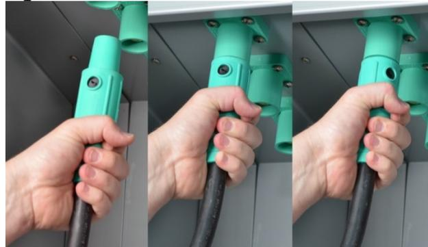
2. Continue with connections, beginning with the rear of the cabinet and working forward
