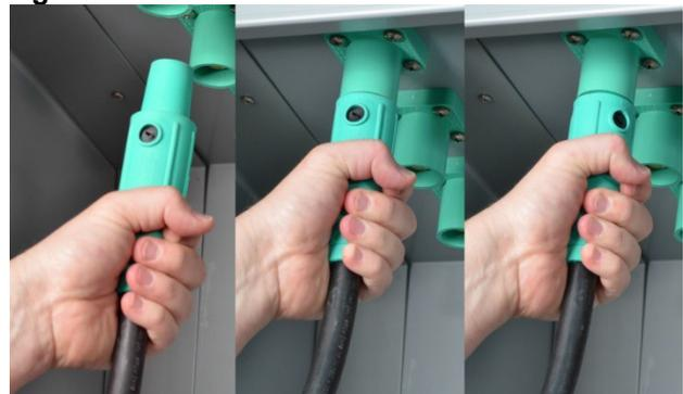
3. Continue with connections, beginning with the rear of the cabinet and working forward
