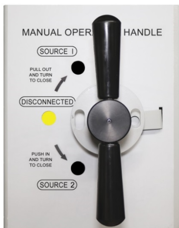
Figure 1. DISCONNECTED (from SOURCE 1) position indicator
