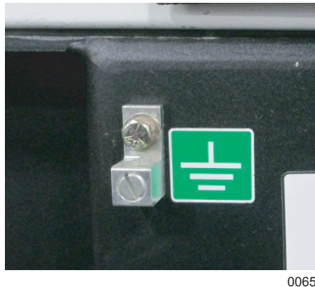
Figure 16 - Frame Ground Connection
